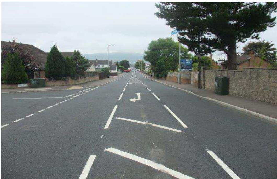
Finaghy Road South – central hatching
